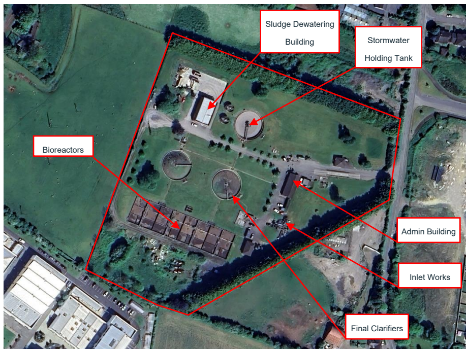
Figure 2-1 – Existing Mortarstown WwTP – Aerial View
