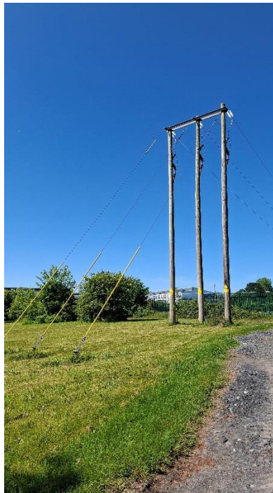
Figure 1-2 - HV 3-Phase Supply into Mortarstown WwTP Site
