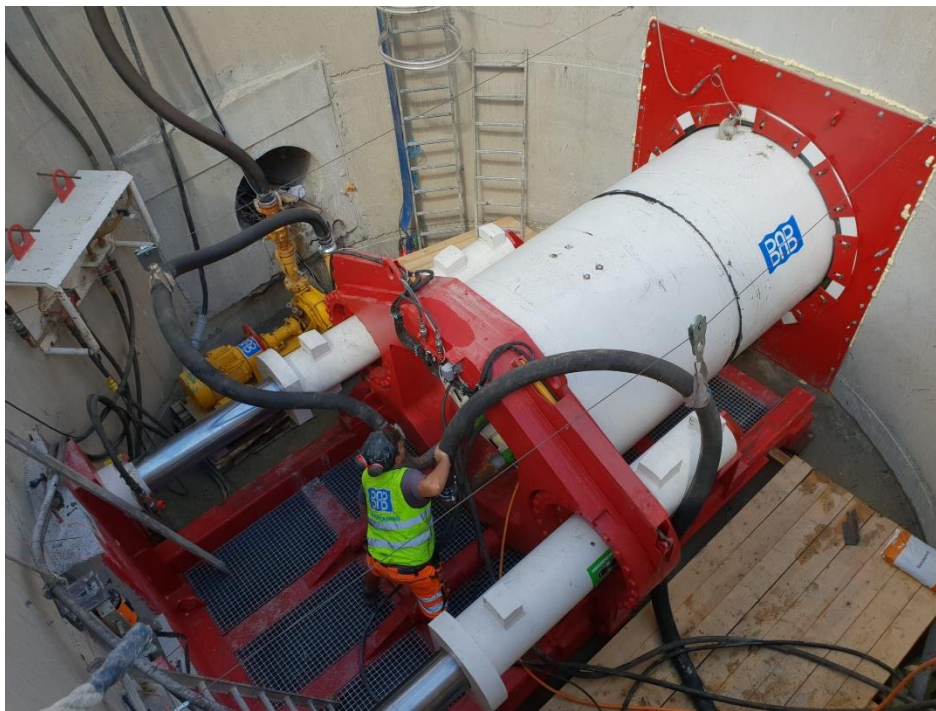
Figure 6 - Example of a compact MTBM jacking operation from a shaft
