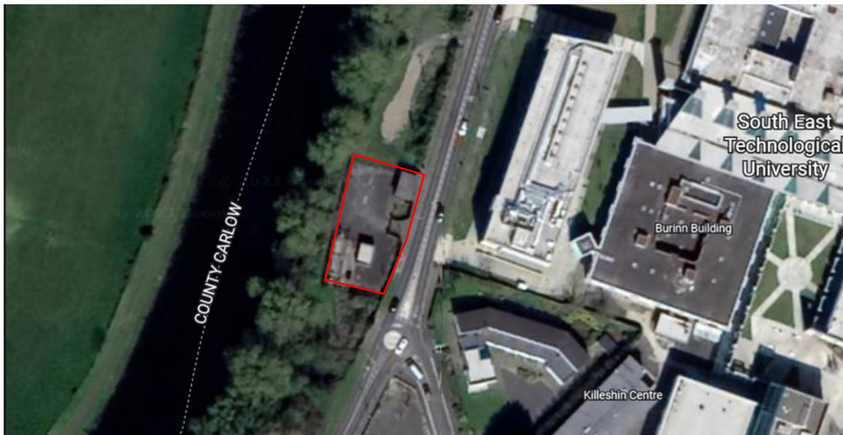
Figure 2-2 – Existing Kilkenny Road Pumping Station – Aerial View
